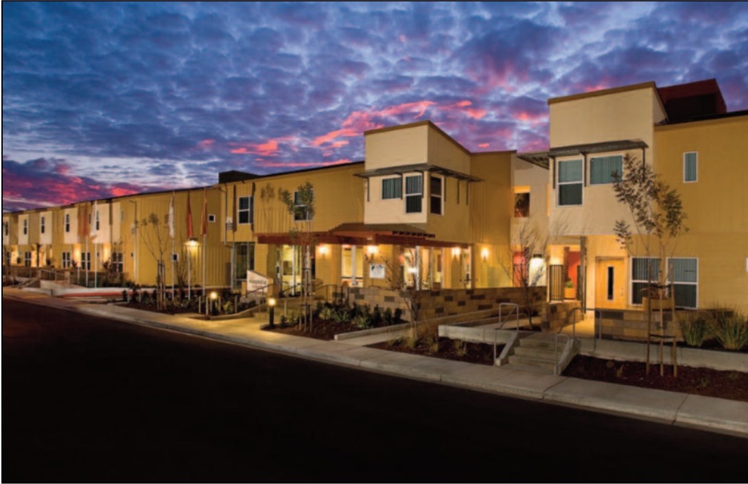
Museum Park 117 Unit Apartment Homes San Jose, CA
